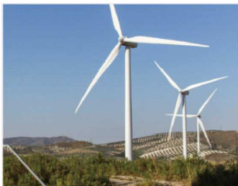
Wind power generation
